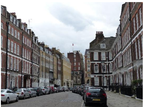
Figure 3 Georgian Housing close to Hyde Park
