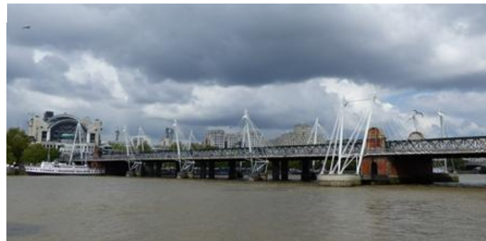
Figure 6 Golden Jubilee Bridge
